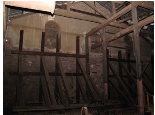
Photograph 4.24 Structural supports to interior of Compressor House
