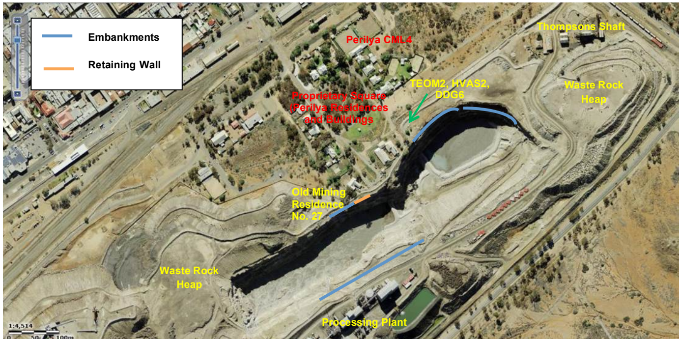
Figure 5-3 Blackwood Pit TSF2 Showing Surrounds
