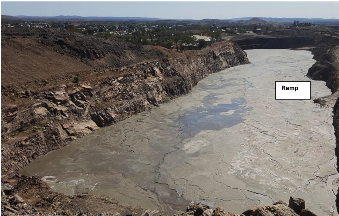
Photograph 10-1 View of Blackwood Pit TSF2, 9 November 2016
