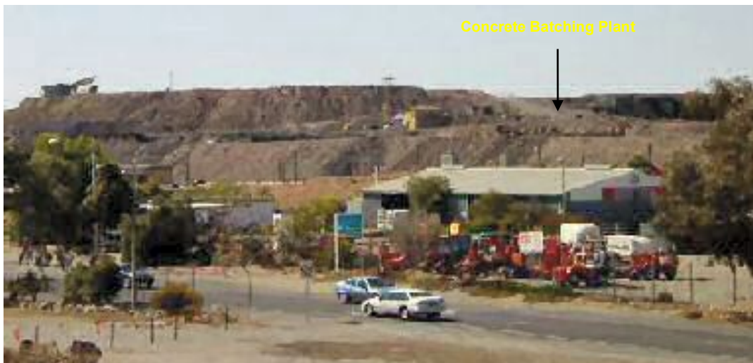
Photograph 5-5 Industrial Sales and Hire Looking to Proposed Concrete Batching Plant
