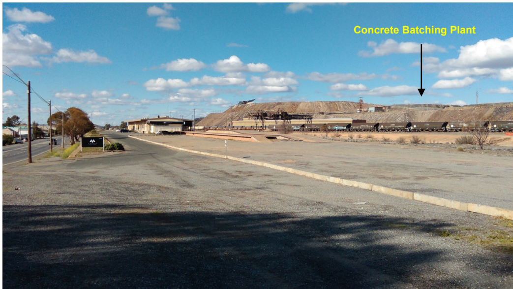
Photograph 5-4 Rail Yards and Commercial Properties Looking East
