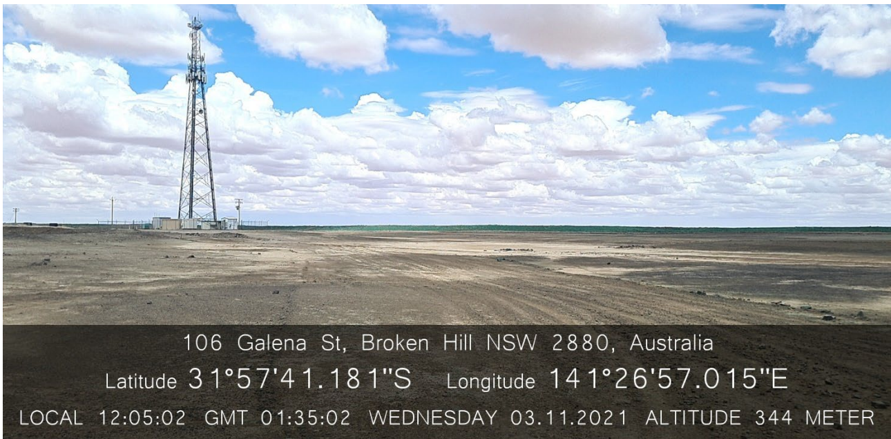
Photograph 1.1 Vodaphone communications tower
