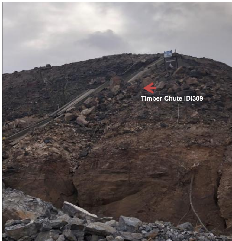
Figure 8-39 Timber Chute ID 308 (I309)
