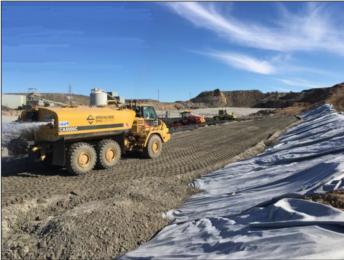
Figure 3-15 Harvesting of Tailings for Fill Platforms During Embankment Construction
