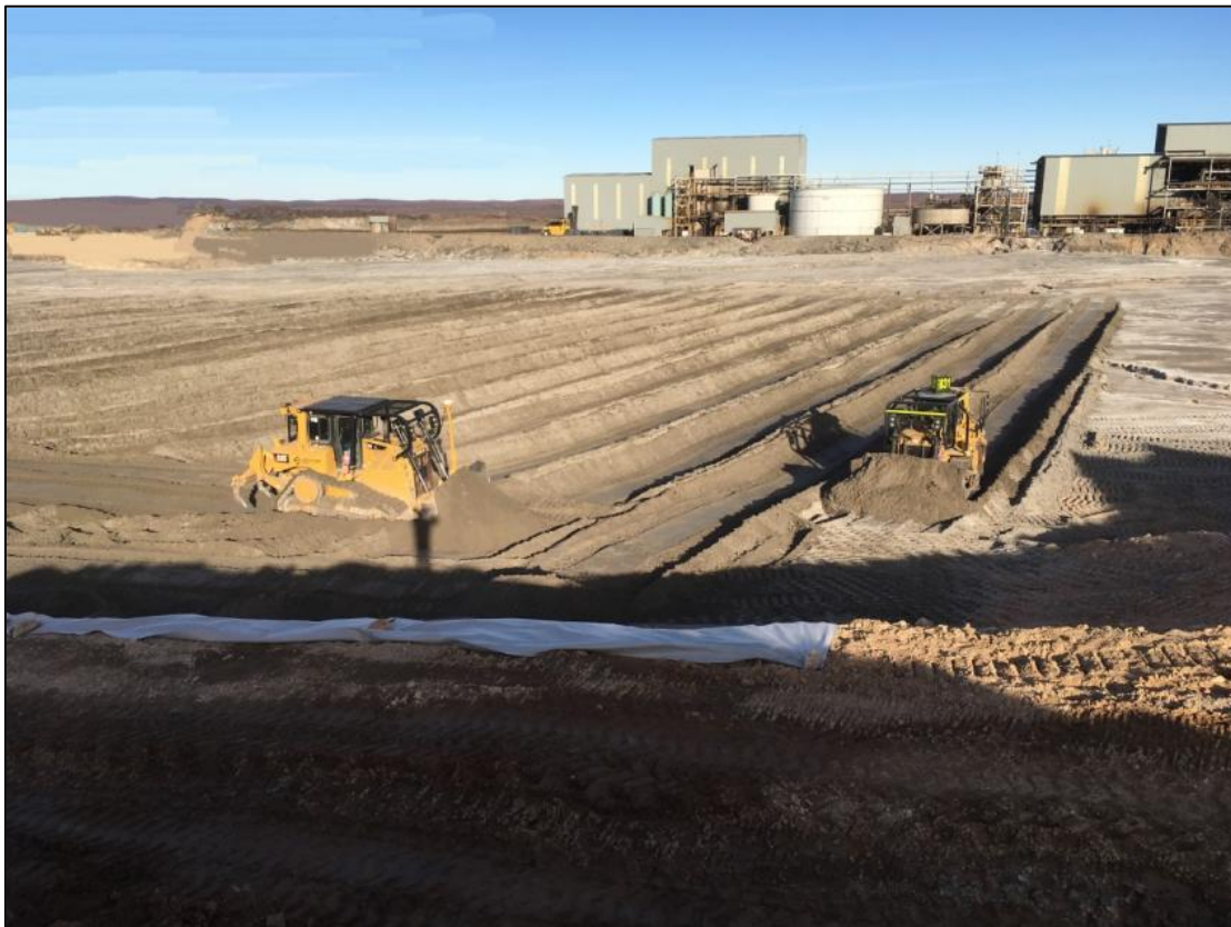
Figure 3-15 Harvesting of Tailings for Fill Platforms During Embankment Construction
