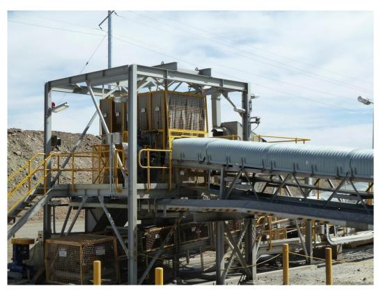
Photo 6. Covered conveyors and enclosed transfer point.
