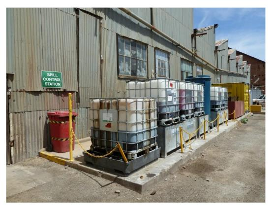
Photo 8. Hydrocarbon storage area with spill kit.
