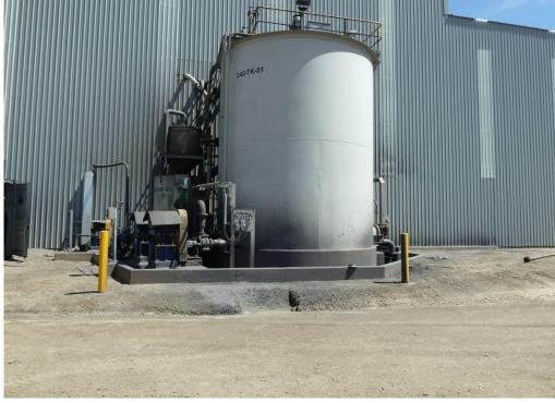
Photo 9. Inadequately bunded lead concentrate tank.
