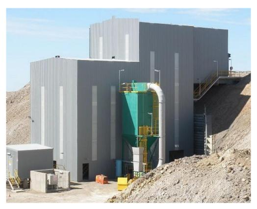
Photo 23. Crusher enclosure and bag house. (Photo by Rasp Mine).
