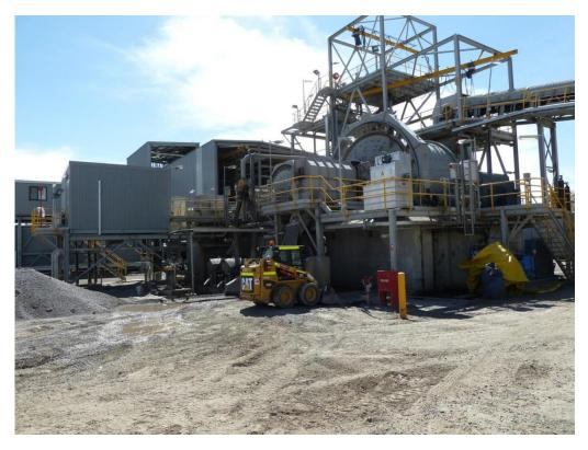
Photo 24. Building installed around the flotation facility providing shielding of the SAG and Ball mills.
