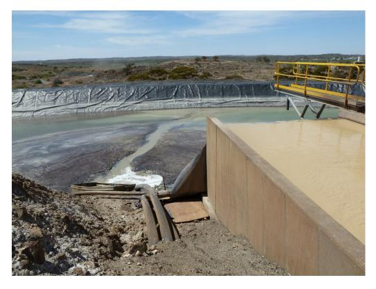
Photo 11. Lined storage pond for water from the water treatment plant.
