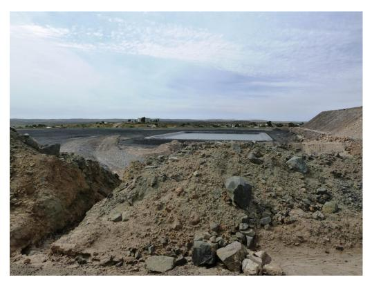
Photo 25. TSF 1 capped with slag and a lined water storage.
