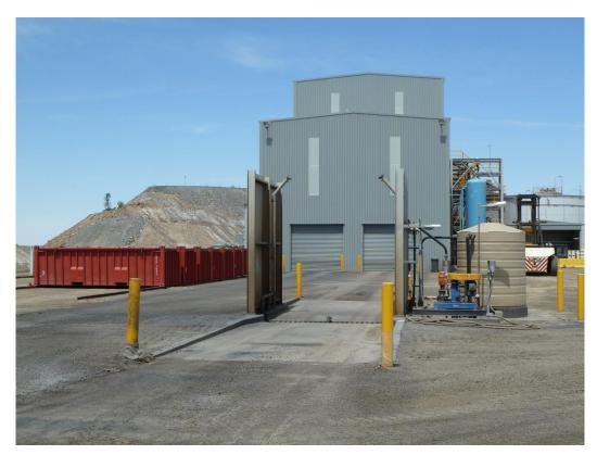
Photo 21. Washdown for trucks and concentrate containers leaving processing plant (in background).
