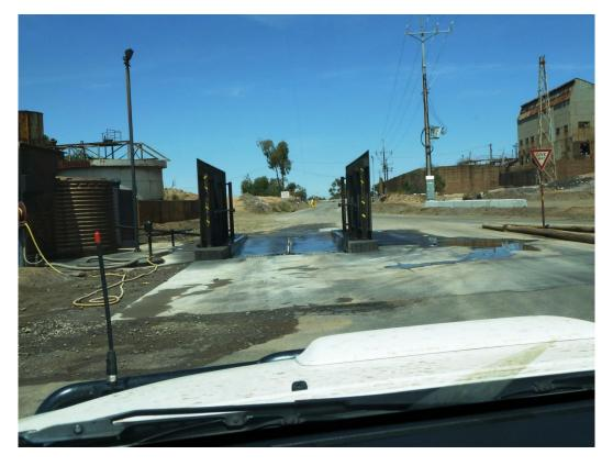
Photo 20. Vehicle washdown at site boom gate.
