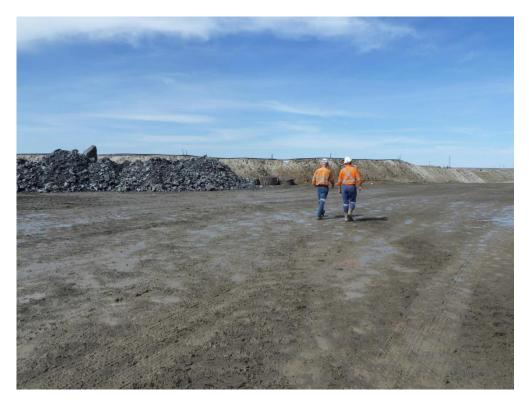
Photo 15. ROM pad showing ore stockpile, bund and water sprays.
