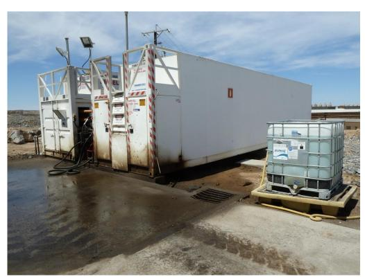
Photo 10. Internally bunded 63,000 litre diesel Transtanks. The sump discharges to an oily water separator.
