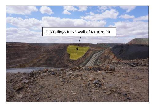
Figure 13- Fill/tailings slope in North Eastern wall of the Kintore Pit
