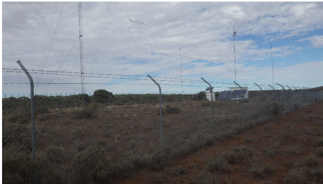
Photograph 15: RFDS radio towers
