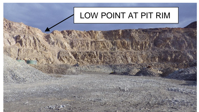
Photograph 14: Kintore Pit, view of southern batter from the top of the waste rock stockpile
