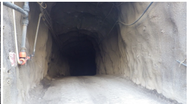
Photograph 20: View down decline from portal
