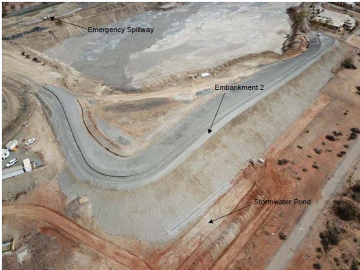
Figure 4-1 Aerial view of Embankment 2, Stormwater Pond and Emergency Spillway
