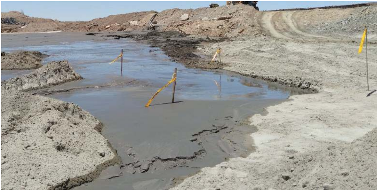
Figure 11 Mill Test Pit After Filling
