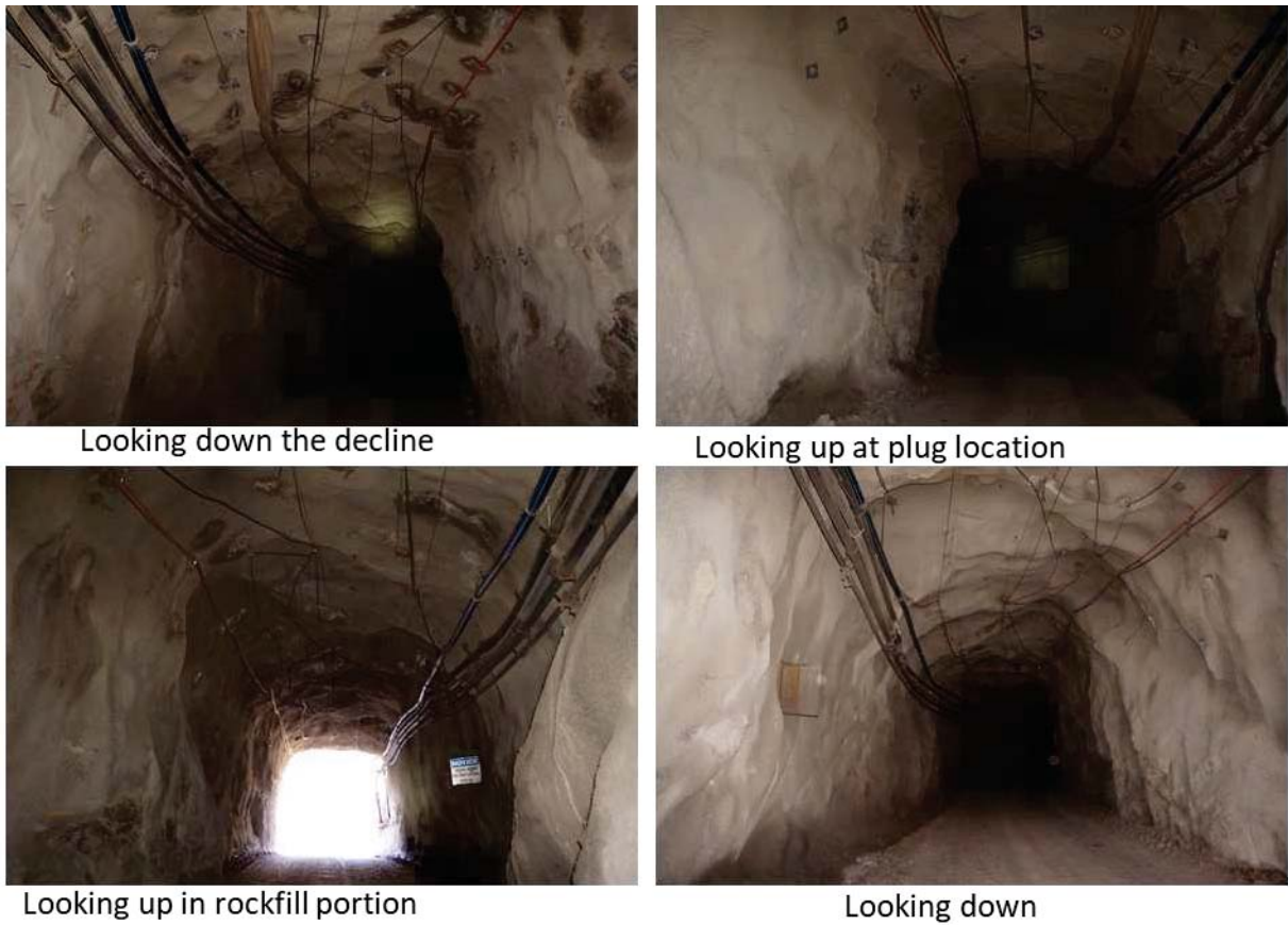
Figure 4: Photos of Portal Plug location
