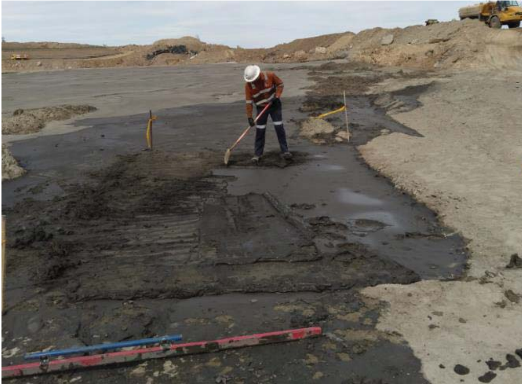
Figure 12 Removing the Zn slurry from the surface of Mill Pit
