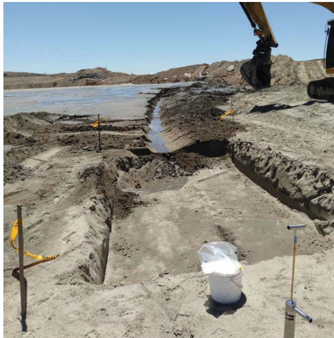
Figure 10 Mill Test Pit Excavated & About to Fill
